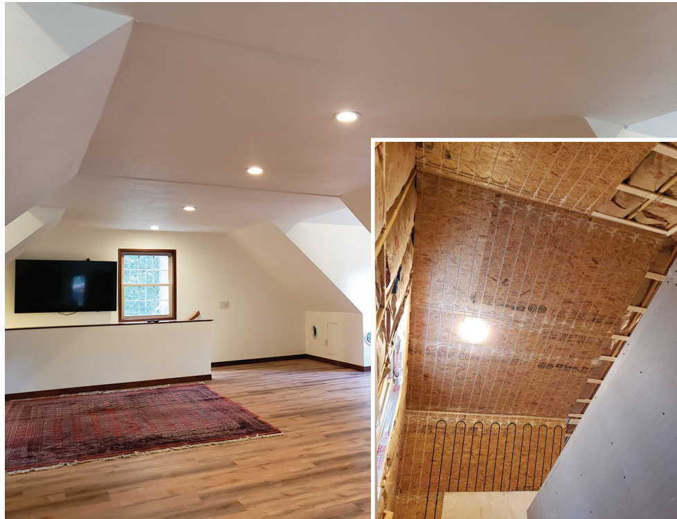
Upstairs plastered Blueboard Heating/Cooling Ceiling. (Inset) Radiant ceiling grid by Hydronics Mfg.
