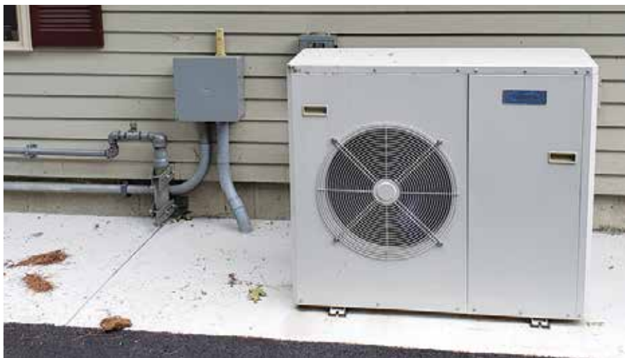
Chiltrix air-to-water heat pump chiller.t
