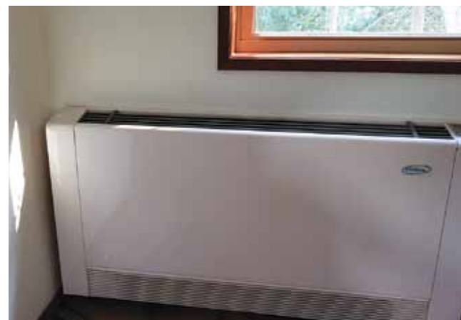
Chiltrix fan coil unit for heating, cooling and dehumidification
